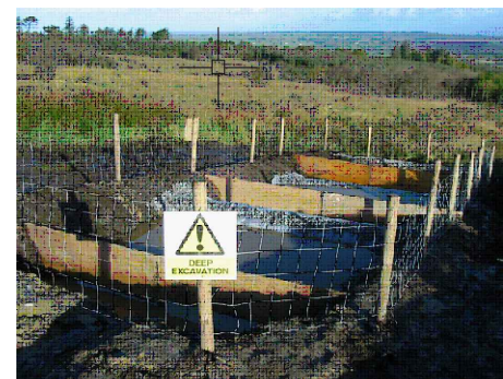
COMPLETED SETTLEMENT POND SYSTEM
